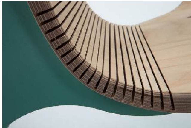
Figure 4.26: Kerf bending plywood chair
